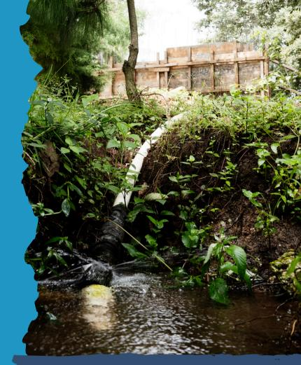
The Panicuy water system will make use of fresh spring water, which is treated and pumped to a holding tank, then fed by gravity to households.
