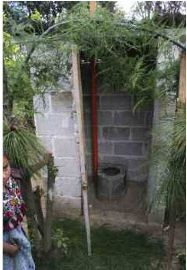
Unsanitary latrines shown in the top photo will be replaced by the vented latrines shown in the photo above. The new latrines are designed to keep flies away and minimize odors.
